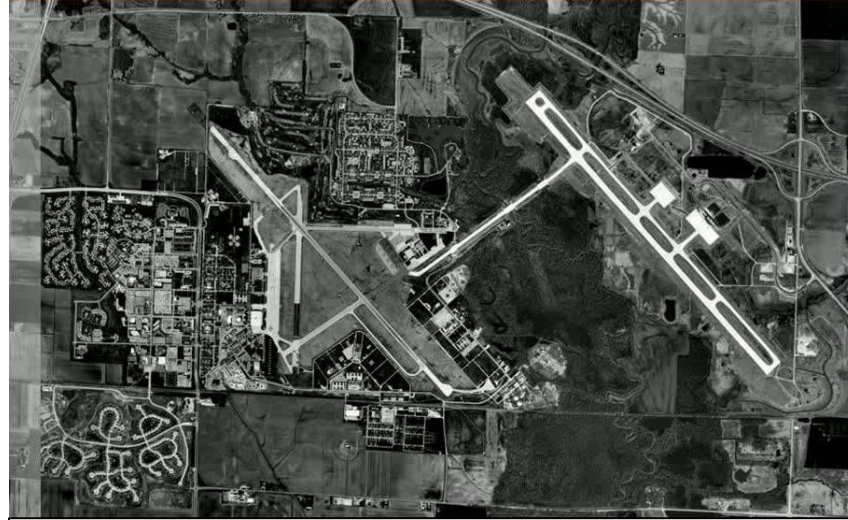
Mid America Airport - St. Louis cargo expansion hopes
